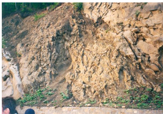
Fig. 7. Megaflow type debris flow – mud flow in Podu Secu Formation in left slope of Buzău Valley, approx. 150 m upstream of the Teherău viaduct.
