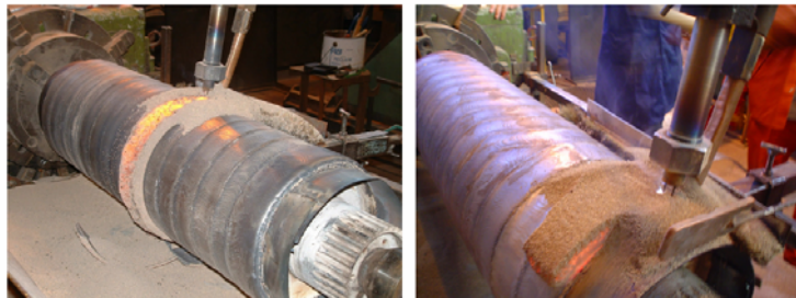
Fig. 10. Procedure 2 – Twin wire welding head 2 x 2.4 mm
