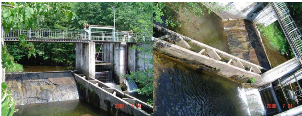
Fig.1. The fish ladder of the Aleu water intake in the Crişul Negru river (source: Crişuri Water Directorate)
