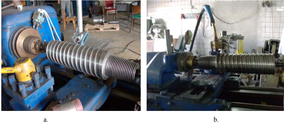
Fig. 3. Positioning and rotating device a. Worm gear fixing; b. Welding head fixing
