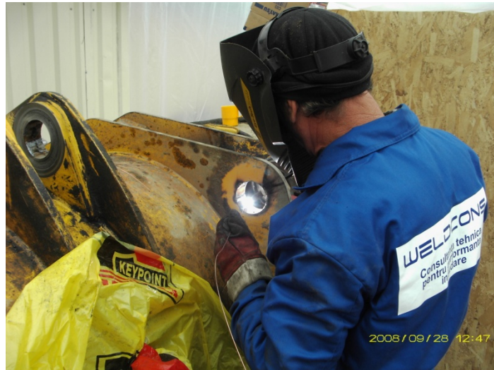
Fig. 9. Rehabilitation by welding a ear bore of bucket
