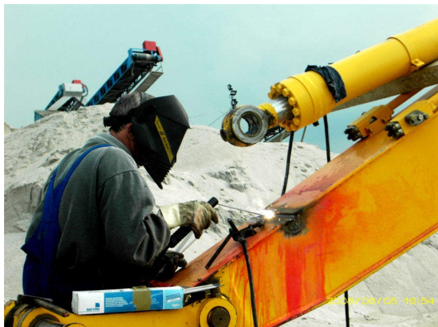
Fig. 4. Welding on excavator arm
