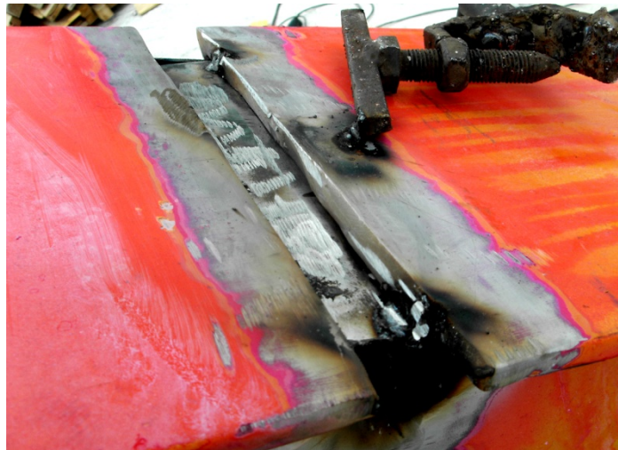
Fig. 3. Fit-up the permanent metallic support and preparing before welding
