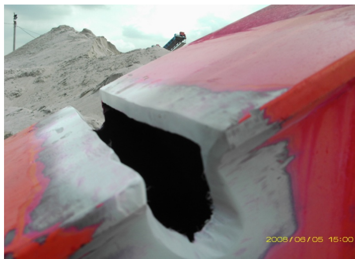
Fig. 2. Penetrant testing after cracks removal
