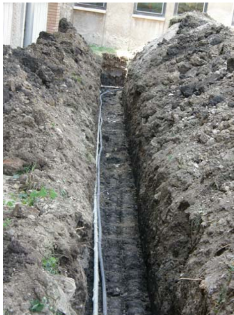
Fig. 2. Black insulated pipe buried at 1 meters
