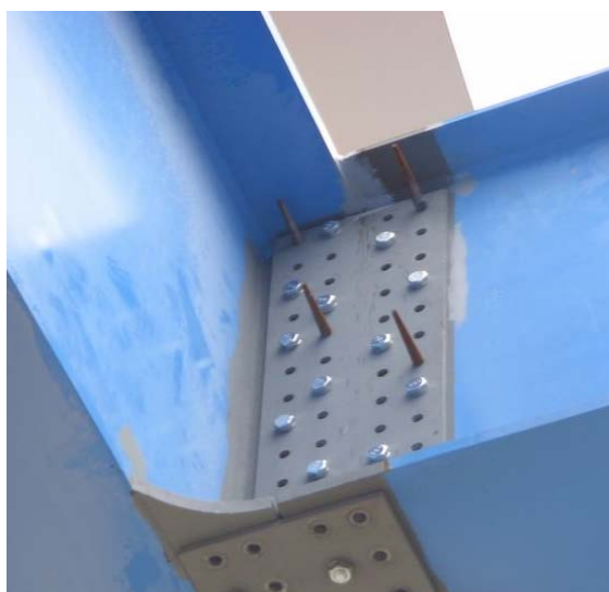
Fig.4. Transversal beams welding
