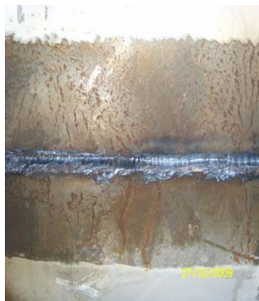
Fig.3. Arc-air roots cleaning
