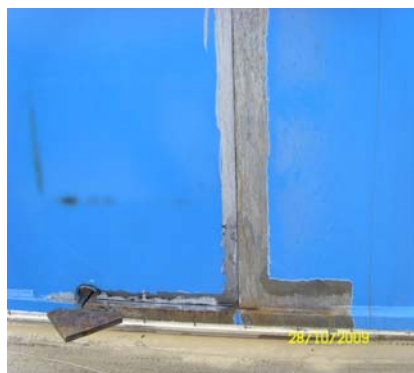
Fig.3. Cuttings-out for soles butt welding
