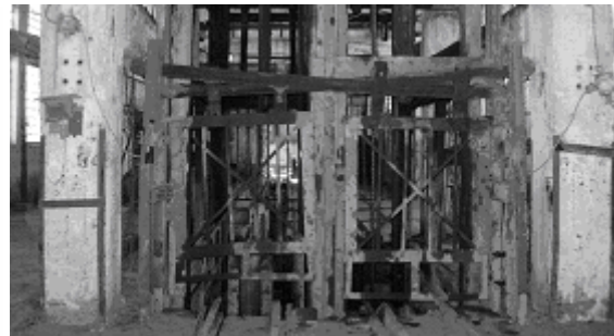
Fig.5. Extraction vessel in ramp
