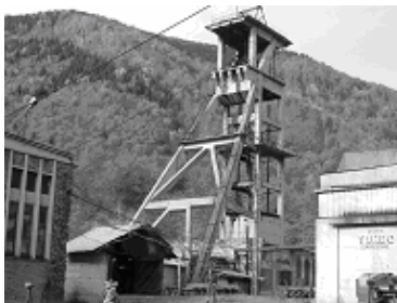
Fig.1. Extracting installation „Auxiliary well Mierleasa“
