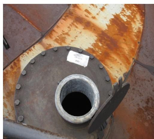
Fig. 2. The holes for taken samples, opened, in direct contact with the atmosphere
