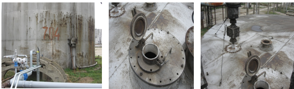
Fig. 10. The tank 704, equipped with a safety respiratory system outdated and inoperative, having the holes for samples taken and for light opened
