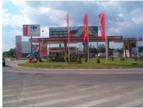
Fig. 1. Terminal (station) for carburant distribution
