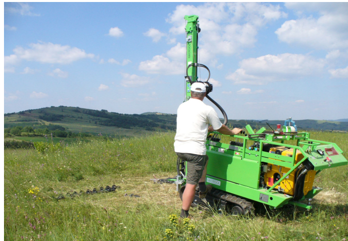
Fig. 2: Aspects related to execution of geotechnical drillings.
