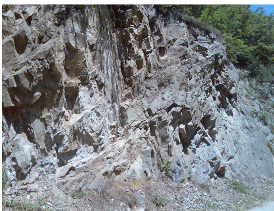
Fig. 1. Outcrop in the igneous intrusion on the slope of Valea Satului river, adjacent road DN 57 Orșova-Moldova Nouă (view from river).
