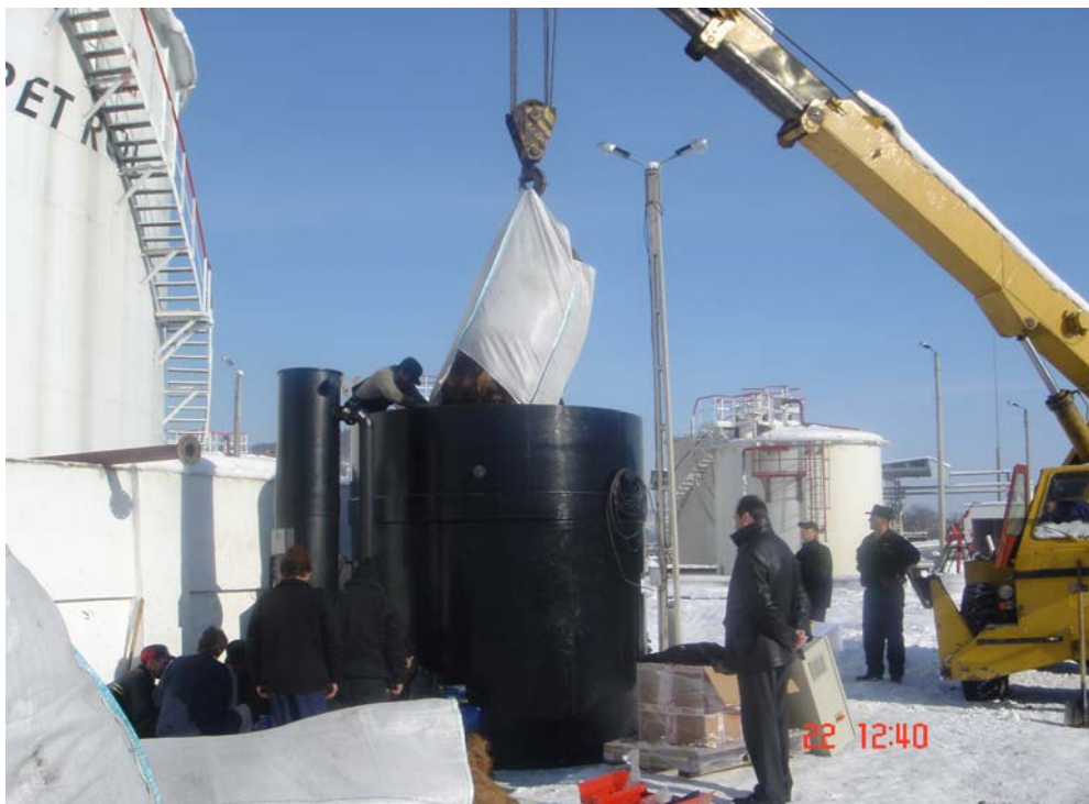
Entering backfill material (Coconut tree bark)
