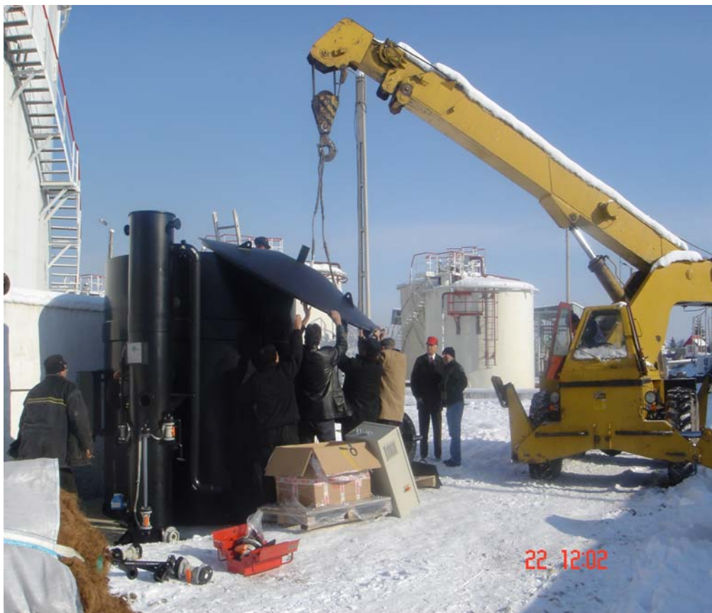
Placing bio-filter in position
