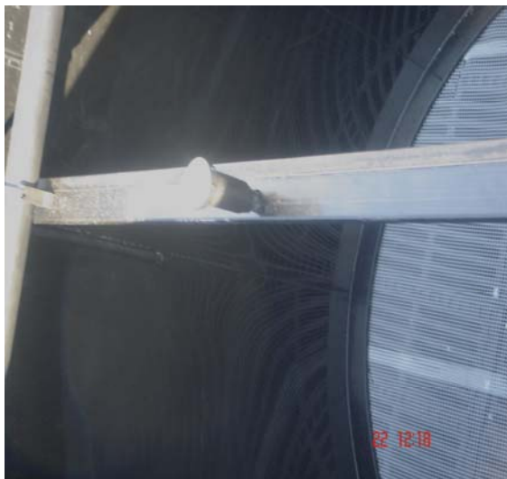
Inside View: Notice metallic holder for filtering mass and automated spraying device
