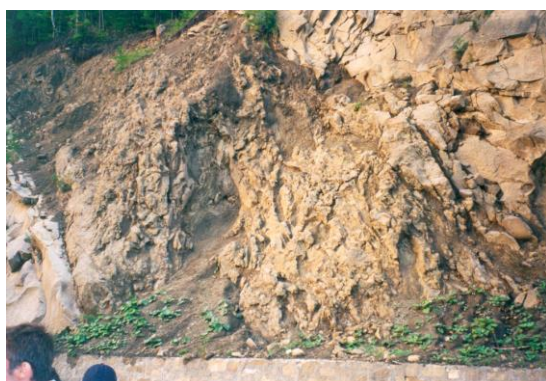
Fig. 7. Megaflow type debris flow – mud flow in Podu Secu Formation in left slope of Buzau Valley, approx. 150 m upstream of the Teherău viaduct.
