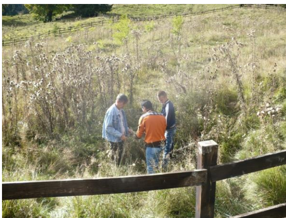
Fig. 7. Drilling in ravine developed at six meters downstream (south-west) to the site
