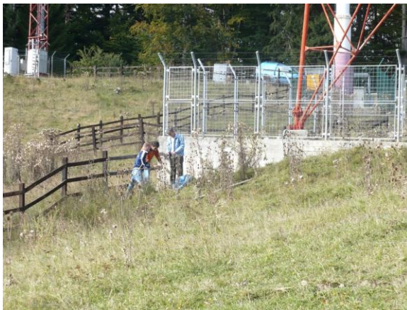
Fig. 5. Drilling in proximal position (south-west) to the tower site
