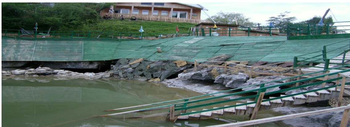
Fig. 8. Overhanging dissolution holes in a horizontal plane – view towards the north-west part of the lake – image taken on July 8 th , 2010
