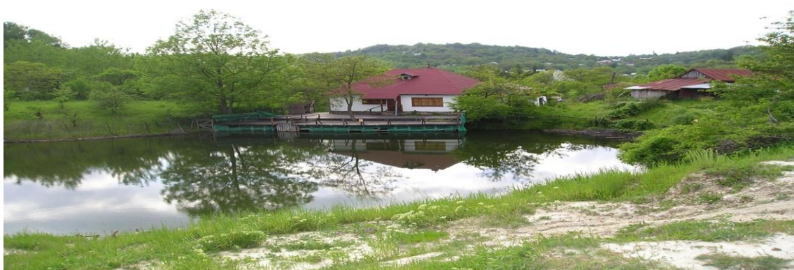
Fig. 1. Upstream slope of the lake“La Butoi” – image taken on May 23 rd , 2014
