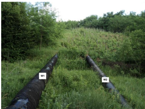
Fig. 2. Old aerial crossing piping line.
