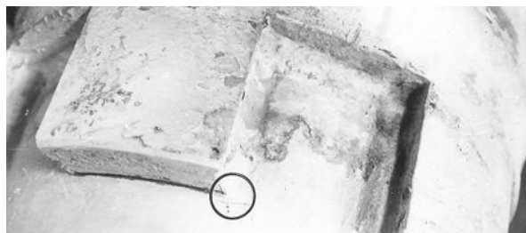
Fig. 5. Drill pipe of 10 \frac{3}{4} in, of series 122: sight of the area with surface fissure
