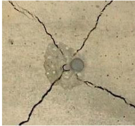
Fig. 13. Radial cracks propagated as a result of the impact of a bullet with a ceramic plate [10]
